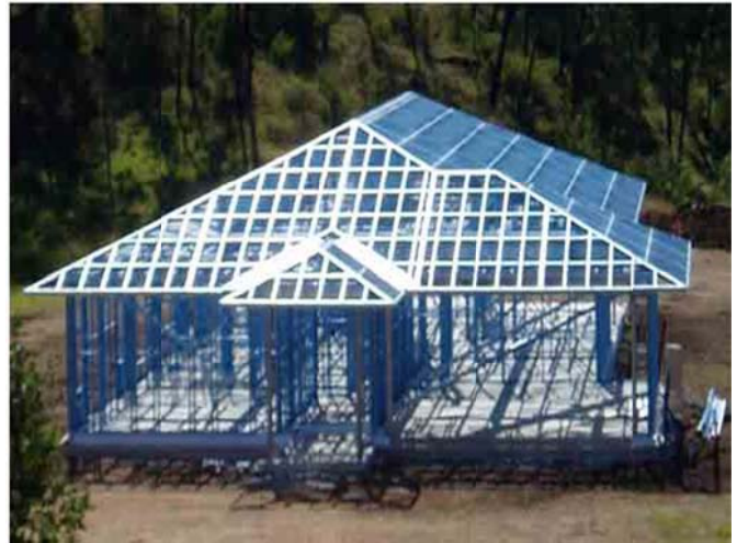
Frames Erected for cladding.
