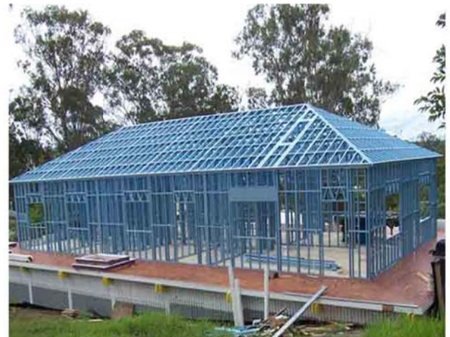
Panelised Steel Frame House.
