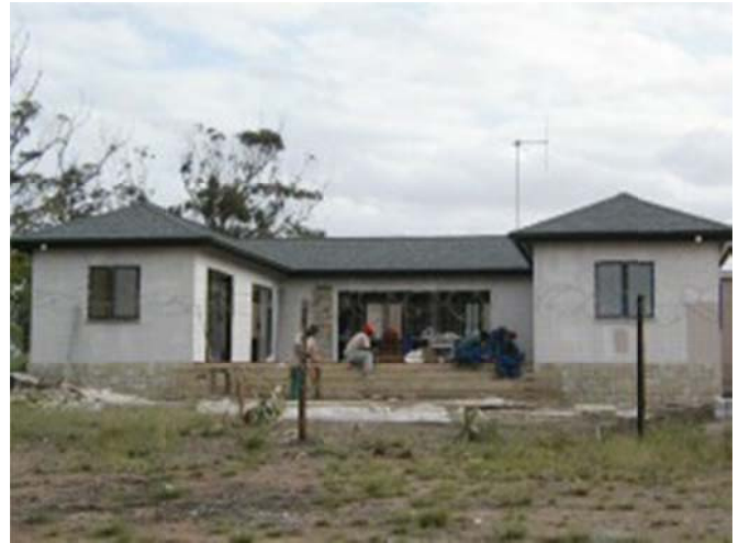
Week 4: House Completed.
