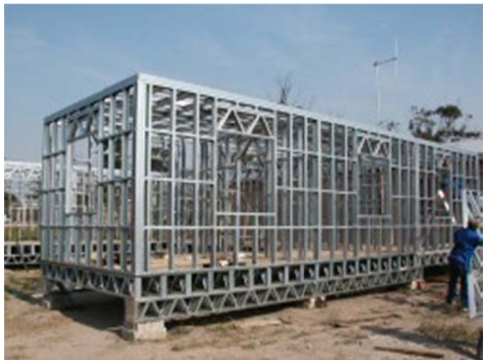
Day Two: Walls & Ceiling Panels Erected
