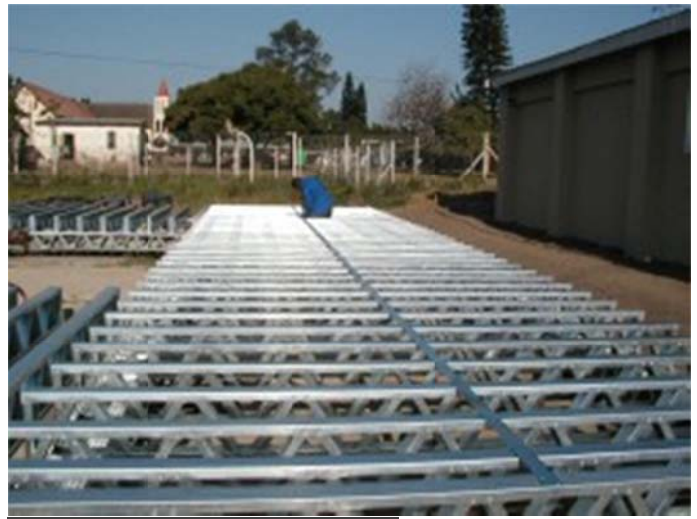
Day One of Project: Floor Joists Installed.
