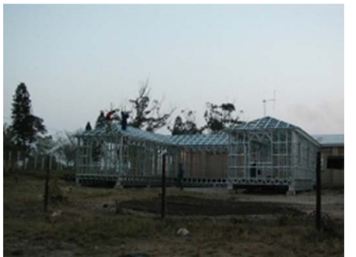
Day Three: All Frames Erected
