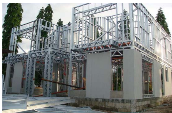
Two storey building using fibre cement board.
