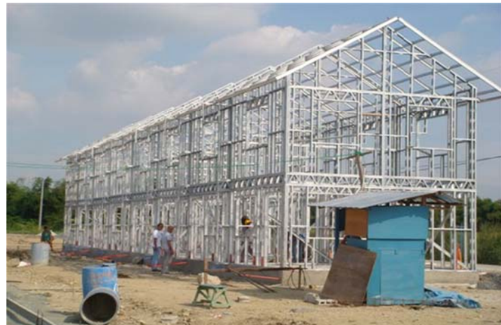
Erected Steel Frame Panels
