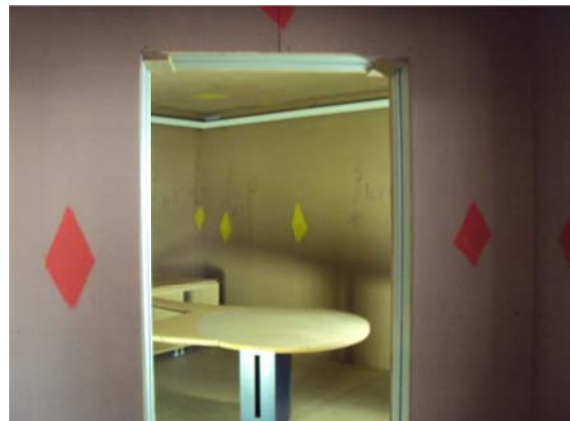
Sound proofed walls.
