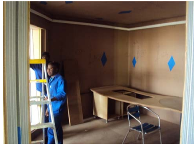
Internal lining of the sound studio.
