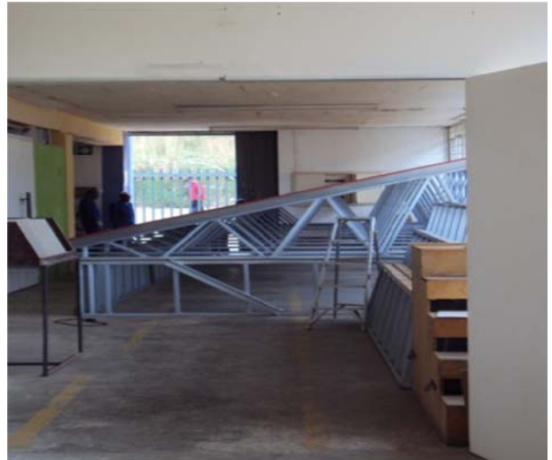
The building being manufactured in the factory.
