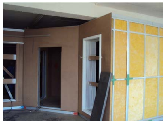
Sound proofing of the studio.
