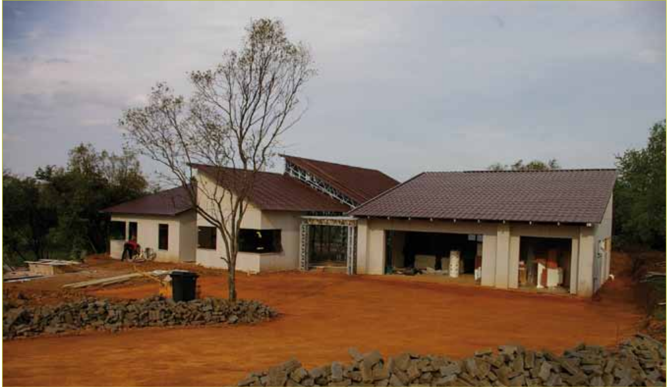
Magaliesburg Bushveld Steel House completed in 12 weeks (Courtesy of InnoSteel)
