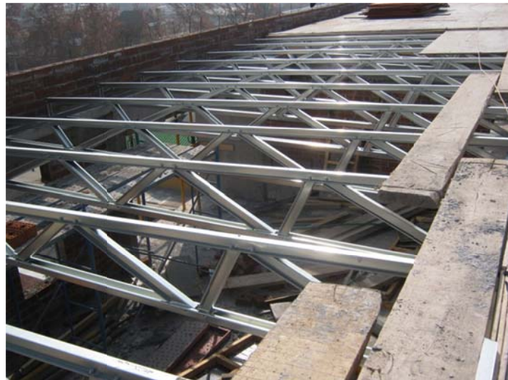
Commercial trusses on a block structure
