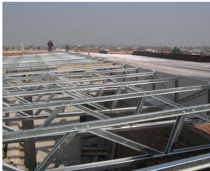
Commercial Trusses Installed Chile.
