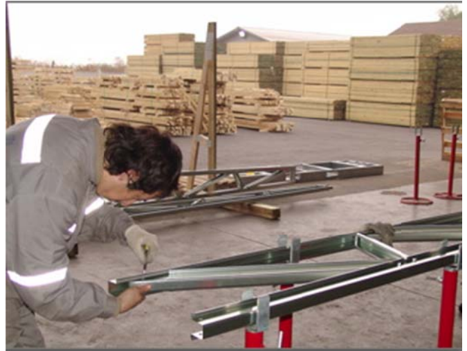
Tecno Truss fabricating steel trusses
