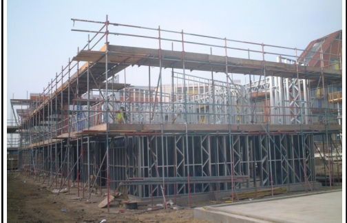
Light steel 140mm profile G380 - load bearing
