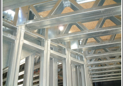
Internal Walls in 90mm profile
