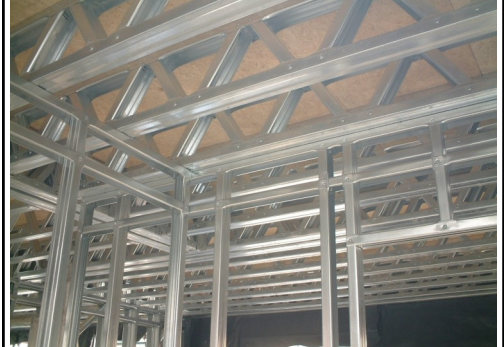
Internal Walls in 90mm profile
