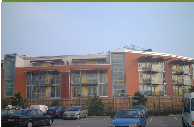
Tile & Rendered facades on light steel frames
