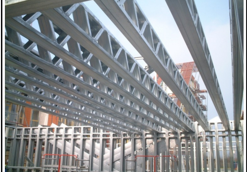
Light steel 140mm G380 sub-floor joists
