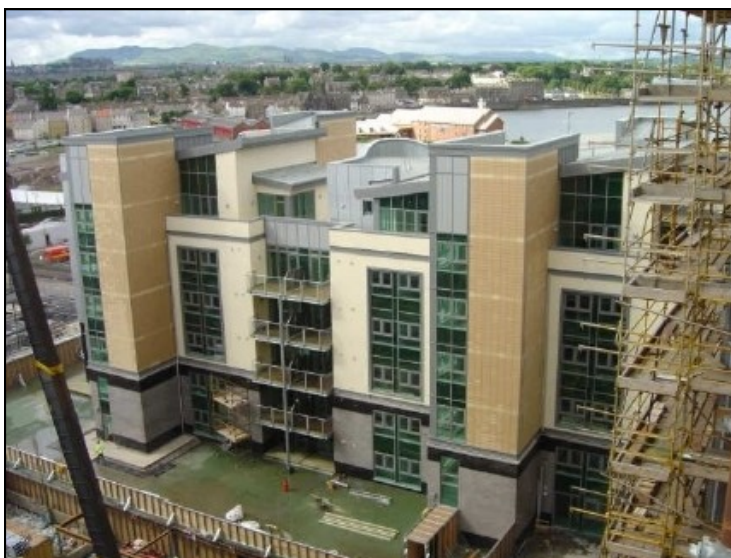
External Rain Screen Framing in Scottsdale 140mm profile and Internal Partitioning in 90mm Scottsdale Profile
