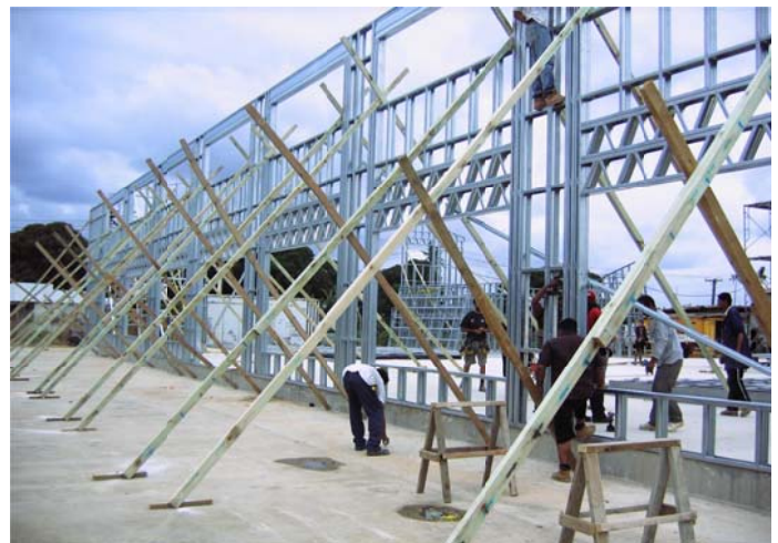
Erection of frames by local labour – Kingdom of Tonga
