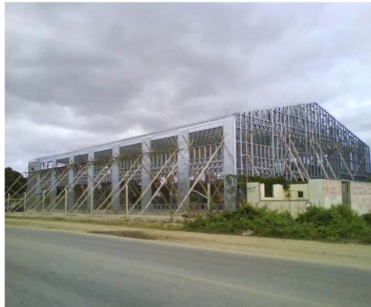
Steel Frame Walls & Trusses erected.
