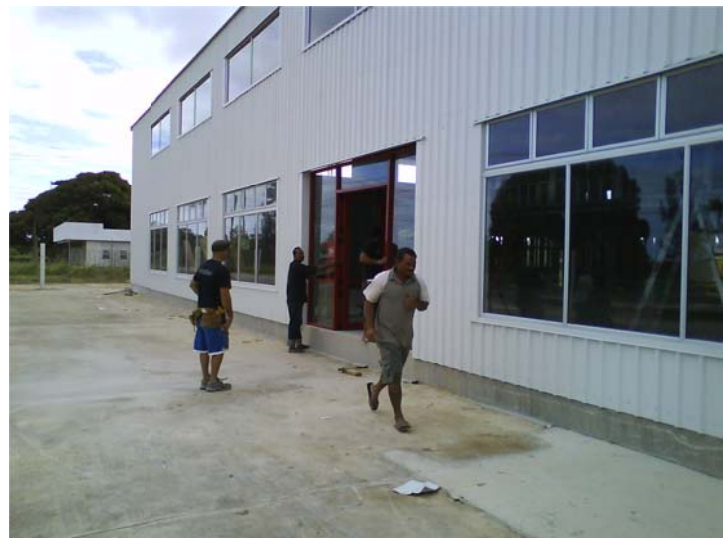
Installation of last windows around the main entrance.
