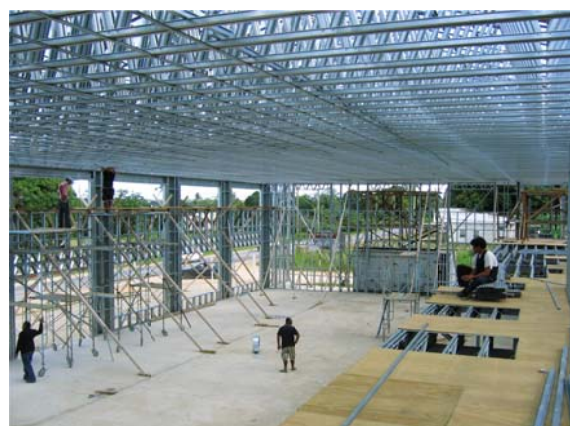
Span capability of Scottsdale's RF600 Truss profile.
