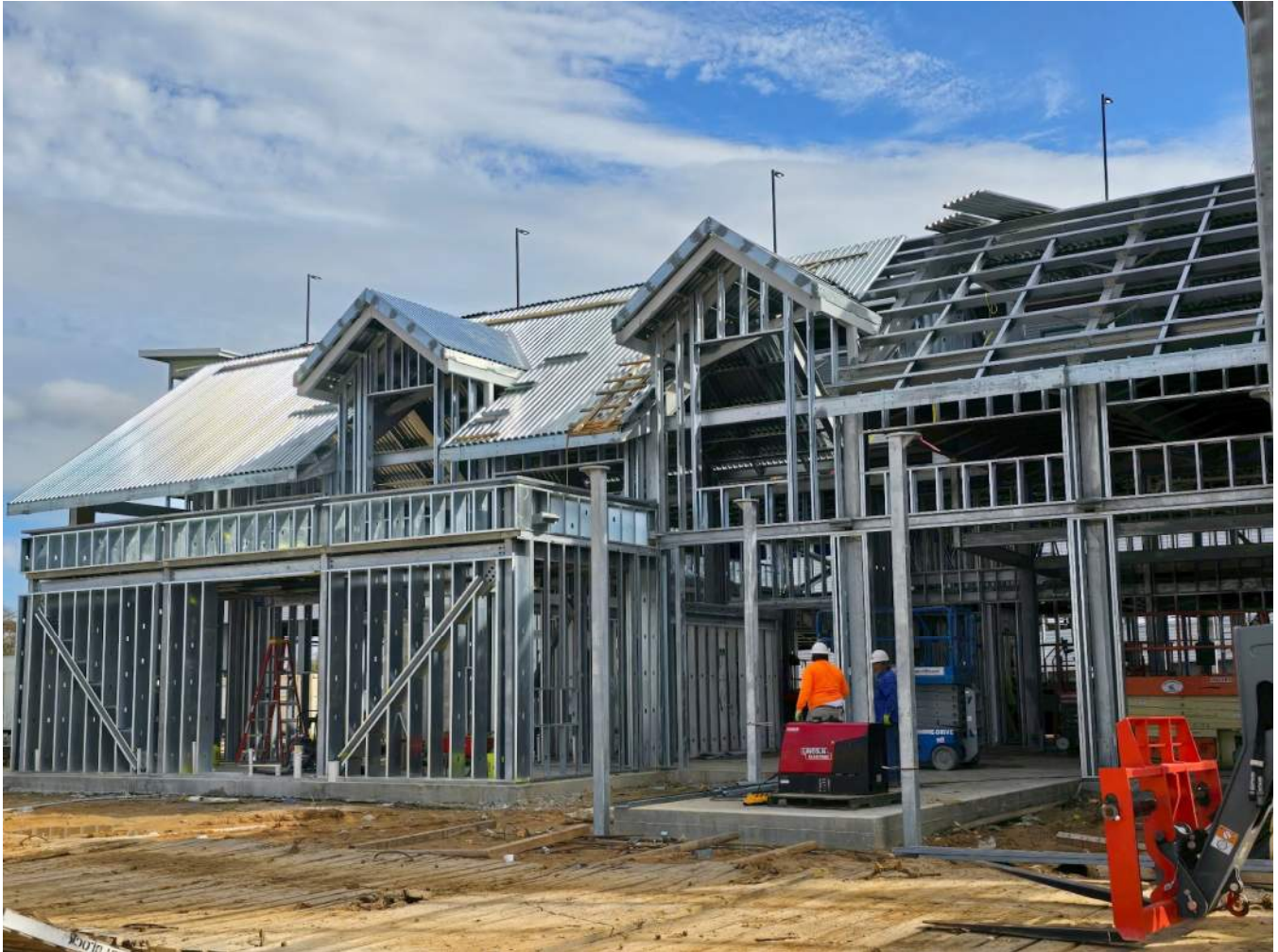
Figure 15 Single-family home construction using KFS Framemaker 1220G3
