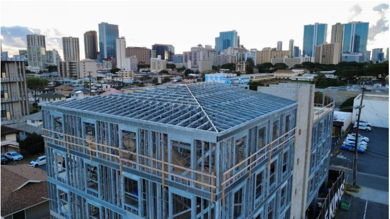
Figure 16 Multi-family construction using KFS Framemaker 1220G3
